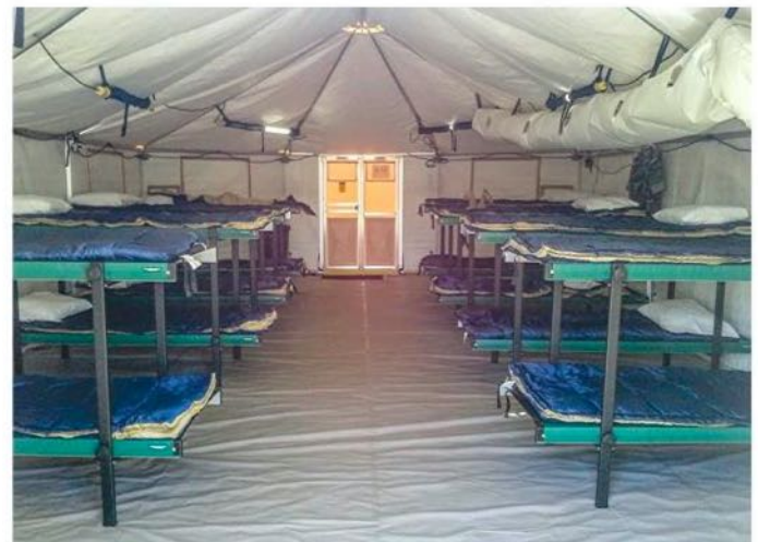
Shelter billering featuring Western Shelter bunk beds, air distribution plenum, lighting and wiring harness.
