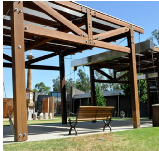
Pergola Structure Recycled Solid Timber Posts Exposed Fixings Timber Type & Colour
