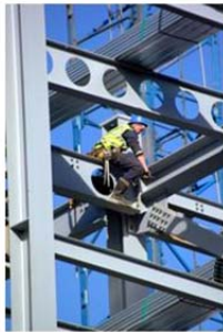
Hot work at heights
