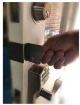
1. Hold the Lock Plate by the tab and slide the plate on the edge of the door from the outside. Close the door.
