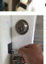
3. Insert the Lock Pin though the Lock Plate into the door frame.
