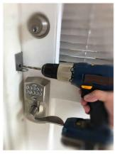
2. Using the guide hole in the Lock Plate, drill a 5/16" hole into the door frame 2" deep.
