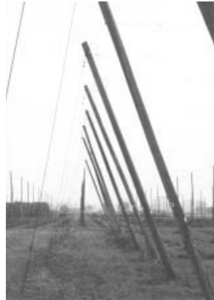
These edge poles in a large Washington hopyard use the same weight cable for both guy lines and cross cables. Cables run both directions from these poles.
