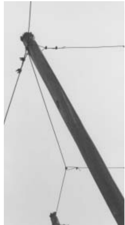
This is an edge pole, with guy line wrapped around the top and fastened with two cable clamps, as is the cable running across the field. The cable parallel to the line of poles is run through the gap between the guy line loop and the pole. Cables between the poles are simply looped around the parallel cable and clamped.
