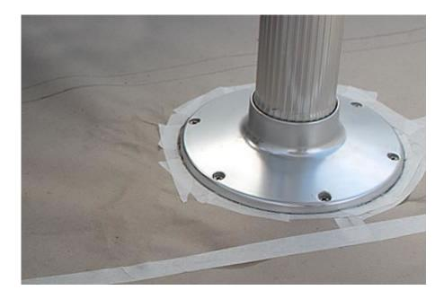
Make a cut from the edge so your finished template can be removed.
