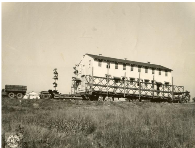
Barracks Building being moved on a trailer, circa 1941. All the barracks buildings were supported by piers and were easy to relocate.
