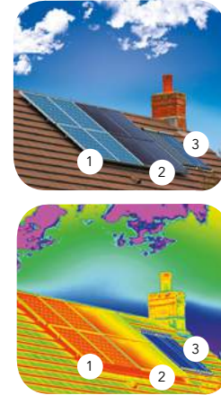
Fig 1. The images above show three types of solar collectors on a typical roof installation: (1) Photovoltaic, (2) flat plate collectors and (3) evacuated tubes. In the thermal image, photovoltaic and flat plate collectors are glowing yellow and red, thus showing they are losing heat, whilst the evacuated tubes are blue showing that no heat is being lost.
