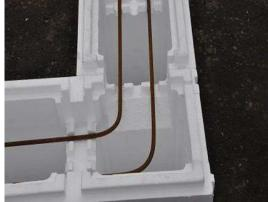
Once the last row of the pool walls has been placed, the blocks can be filled with concrete. The maximum rise speed is 75 cm / hour. Flatten the top of the wall with a circular motion. Bear in mind the possible profile for the liner. Excess EPS parts can be cut off.
