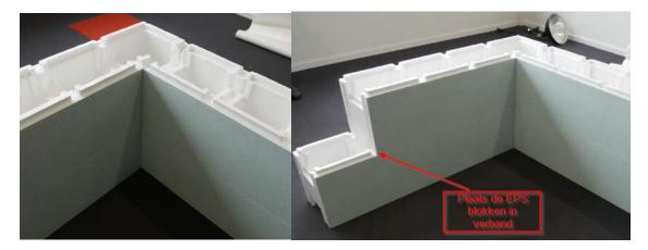
Insert reinforcing steel  $1 \times 10$  mm in each row. In the third row, we recommend  $2 \times 10$  mm horizontal reinforcement. These must be at right angles to the vertical reinforcement.
