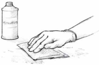
Figure 6 Clean the surface. Use a solvent, if necessary, to remove all contaminants.
