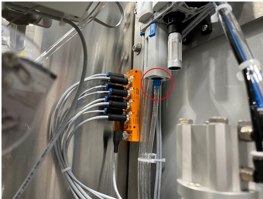
Fig. 1: Filter Drain Location.
