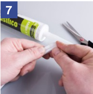
7 Clean off the excess silicone and leave for about 1 hour to dry. Drying time depends on the type of silicone used.
