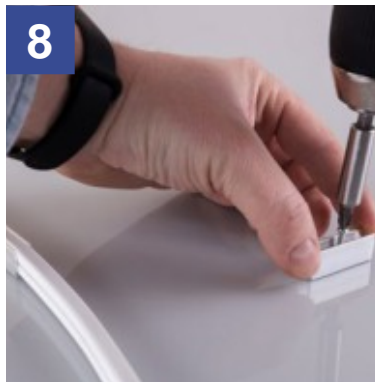
8 While silicone is drying, you can install mounting brackets or mounting profile in planned installation spots.
