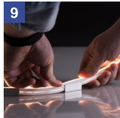
9 Once the silicone is dried and the mounting brackets are in place, press the Neon Flex into the prepared installation spot.
