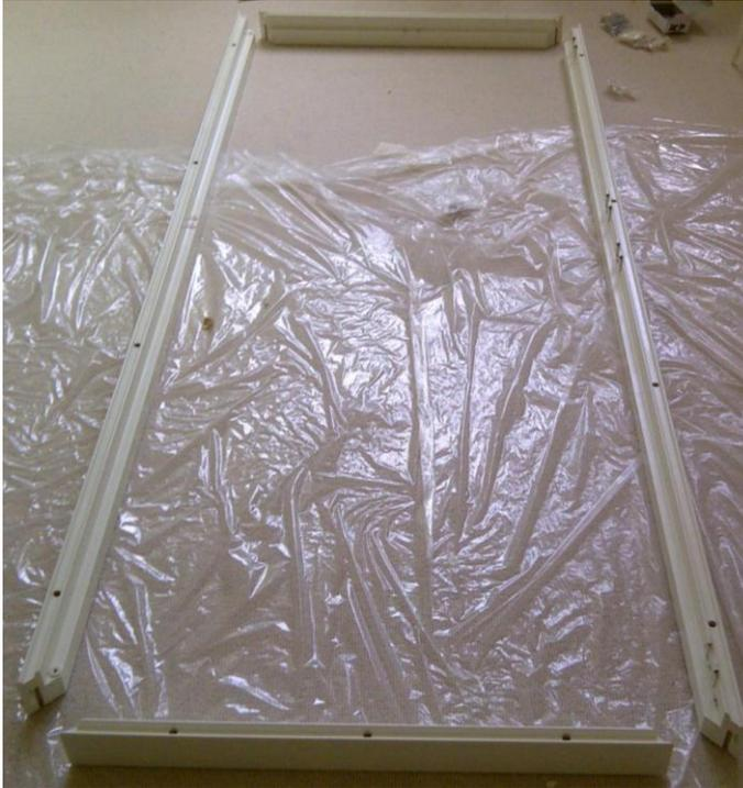
2. Assemble the shutter frame by inserting a nylon 'Hoffman key' (found in the hardware box) into each corner joint. *Remember that if the shutter set is CAFÉ STYLE, the horizontal frame profile will be at the bottom rather than the top.* If using a deco frame, each corner is also secured by a diagonal screw for added strength.
