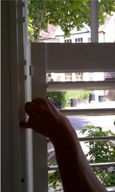
12. If using the frame with insert strips, refit the strips to hide the screw heads.
