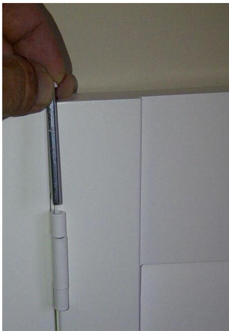
9. Hinge the second panel to the first and so on until all the panels are fitted. If fitting a tier on tier shutter set, the upper and lower panels can be identified by looking at their backs. The upper panels will have the magnets fitted at the top of the panels, whilst the lower panels will have them at the bottom. The lower panels will also be fitted with panel feet, whilst the upper panels will not.
