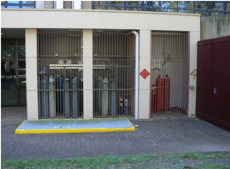
Figure 8 Example of a bulk storage location for cylinders at UOW Wollongong Campus
