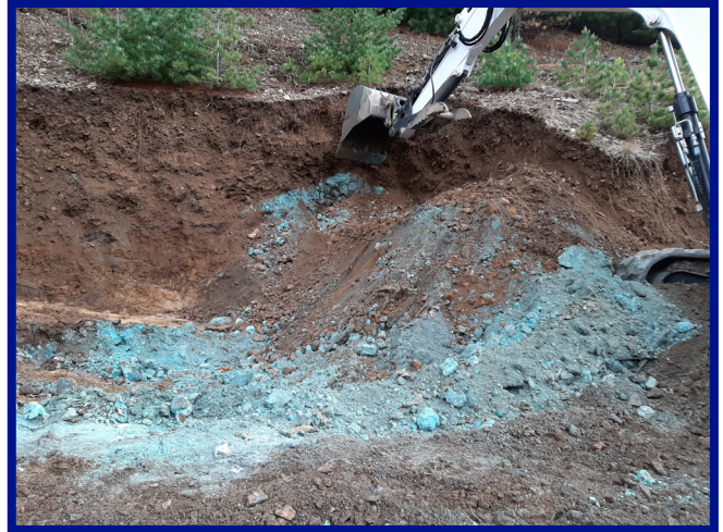
Copper flue dust reserves from the Bunker Hill Lead Smelter found near Kellogg. This is extremely high in lead, cadmium, arsenic, and mercury
