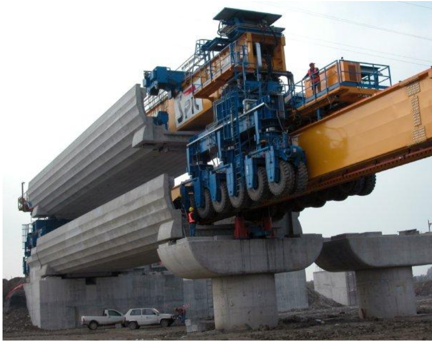
Figure 35: Carrier moving forward along a 78m, 218ton underbridge
