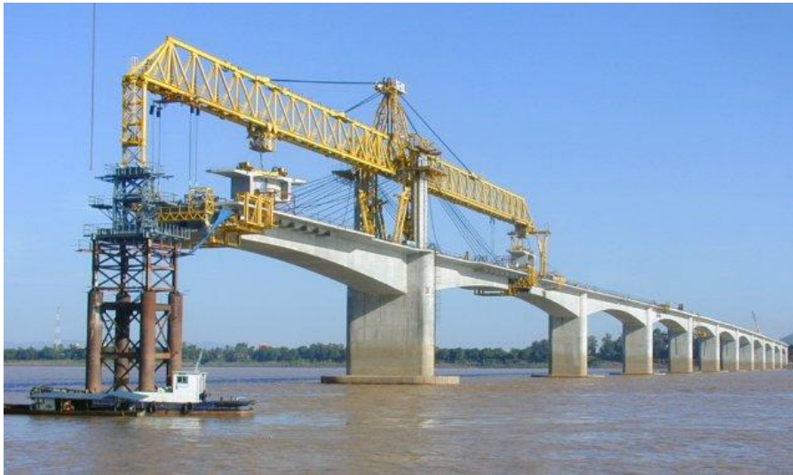
Figure 25: 160m, 320ton gantry for 102m spans and 105ton segments (VSL)
