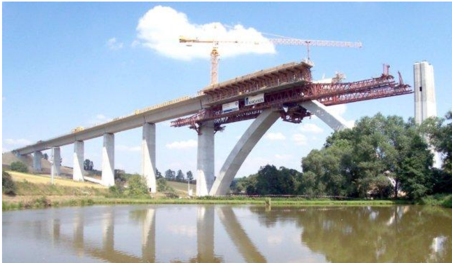
Figure 14: 97m, 690ton underslung MSS for 44m, 1190ton dual-track HSR spans (ThyssenKrupp)
