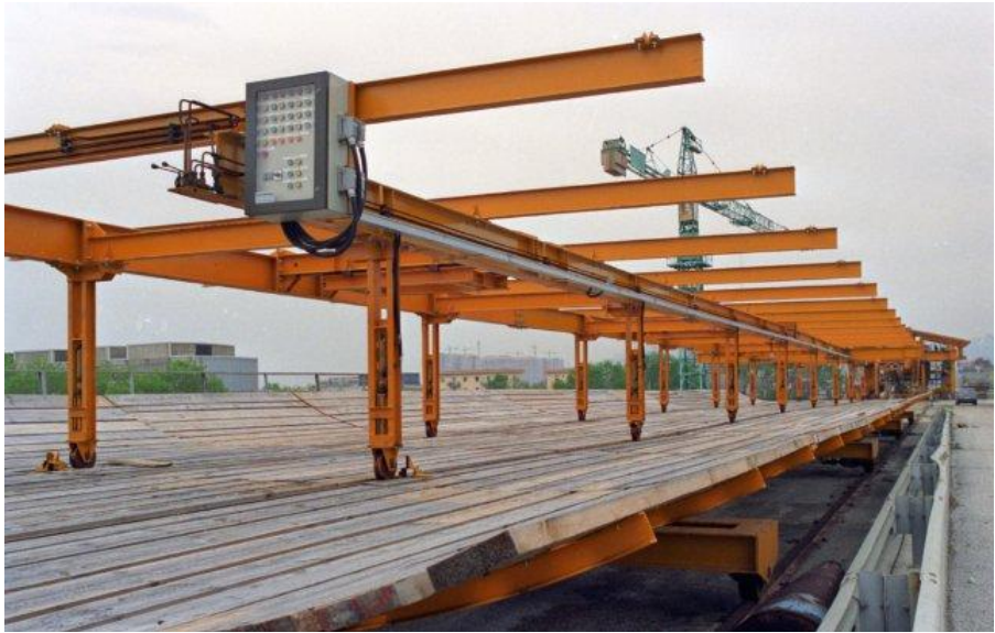
Figure 19: Cage carrier for 47.5m spans
