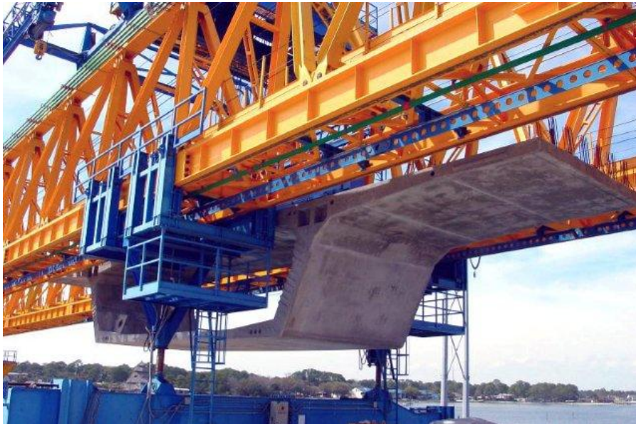
Figure 4: Longitudinal movement of the segment (HNTB)
