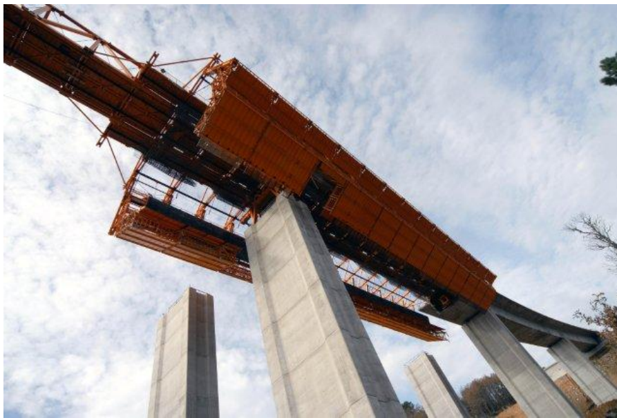
Figure 17: Opened outer form during launching (AP Bridge Construction Systems)
