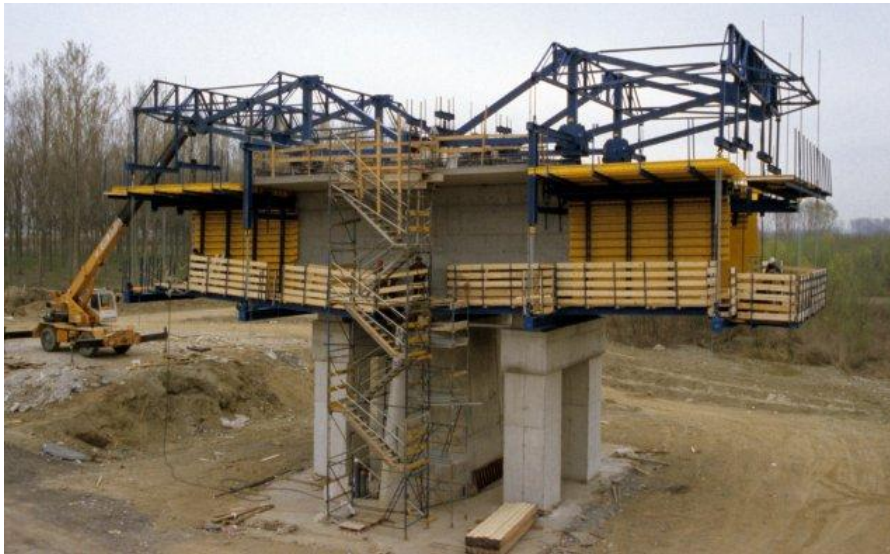
Figure 28: Overhead form traveler
