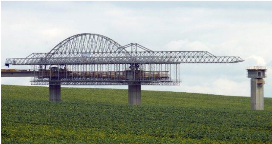
Figure 21: 140m, 780ton overhead MSS for 70m, 1400ton spans (BERD)
