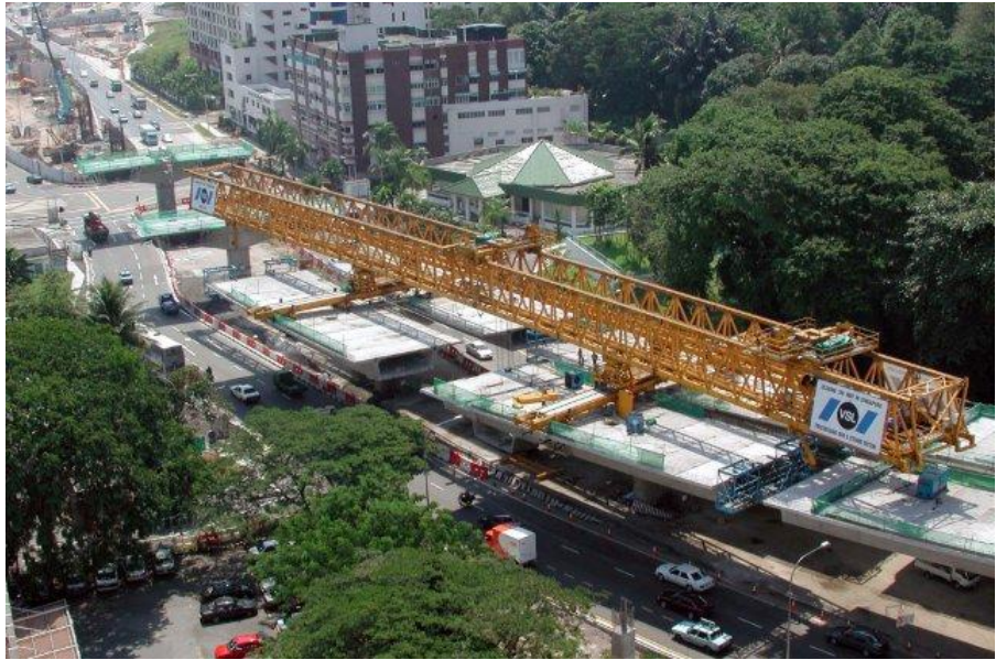
Figure 26: 108m, 278ton gantry for 45m spans and 60ton segments (VSL)
