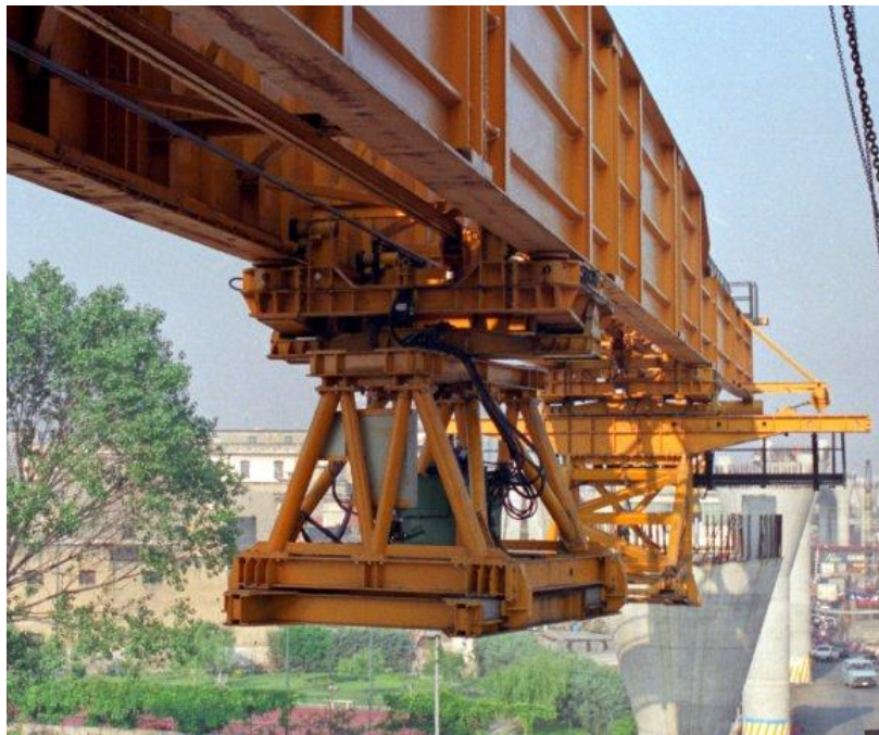
Figure 10: Friction launchers suspended from the main girder
