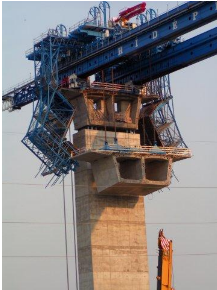
Figure 33: Strand-jacking of 8.0m, 650ton segment (ThyssenKrupp)
