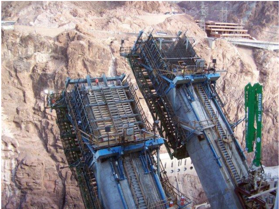
Figure 31: 18.7m, 122ton underslung traveler for 7.9m, 267ton arch segments (NRS)
