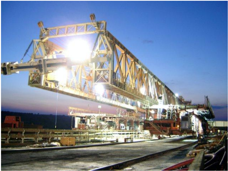
Figure 6: 46m casting cells for midspan (left) and pier-head (right) macro-segments
