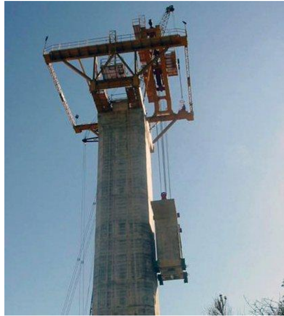
Figure 23: Lifting of 90ton pier-head segment (Comtec)
