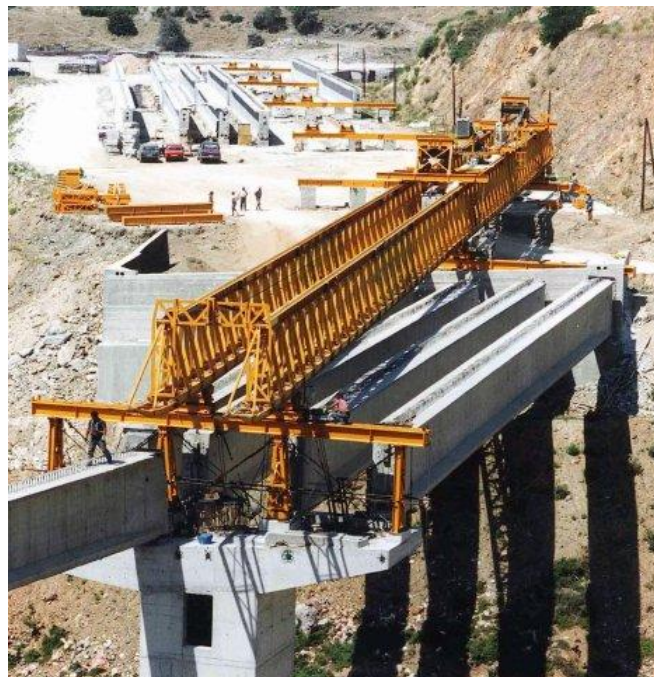
Figure 1: 102m, 90ton launcher for 45m, 120ton beams (Comtec)
