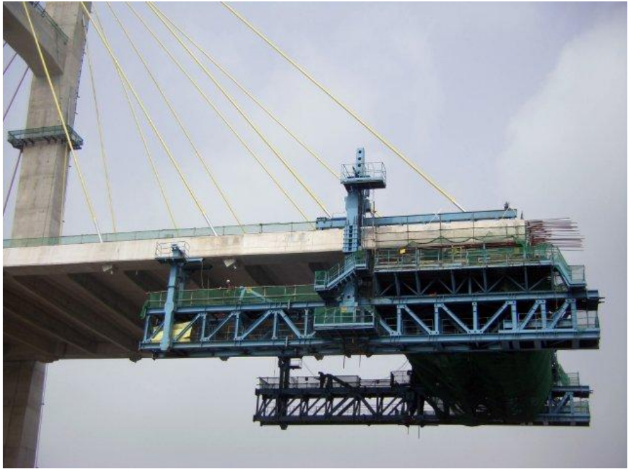
Figure 30: 24m, 202ton underslung traveler for 9x24m, 320ton deck segments (VSL)
