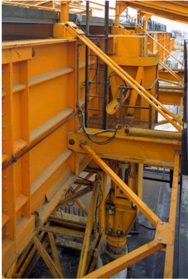
Figure 18: Front support leg
