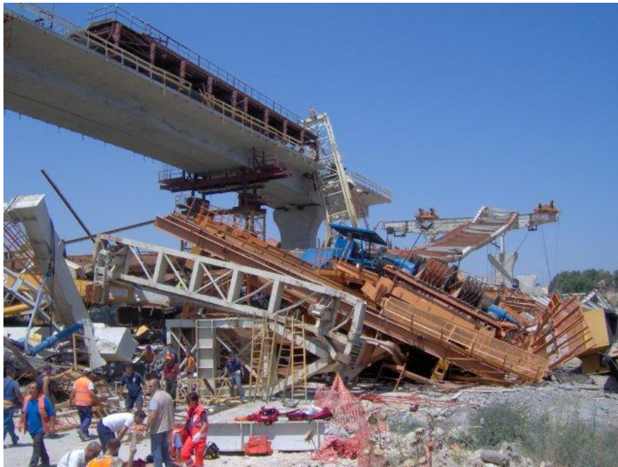
Figure 43: Gantry collapse
