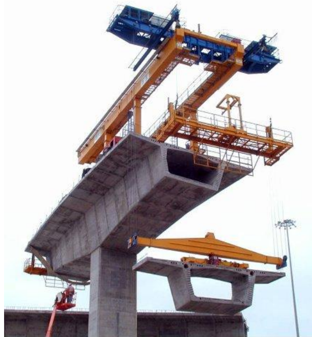
Figure 24: 30m, 90ton lifting frame for 64ton segments (Deal)
