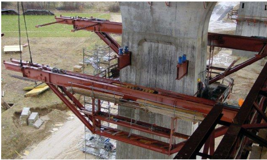
Figure 38: Dismantling of a W-frame on through girders
