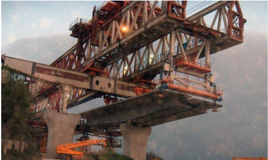
Figure 5: 46m, 640ton pier-head macro-segment placed with a 162m, 1280ton overhead gantry
