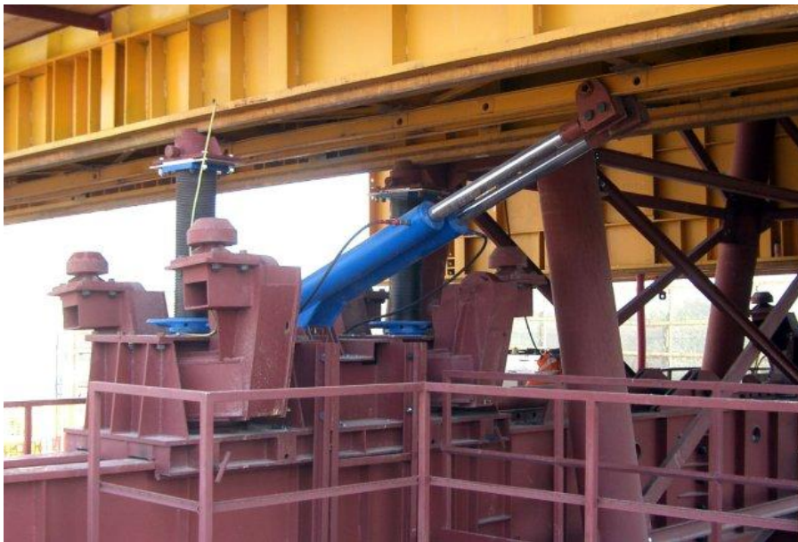
Figure 8: Launch cylinders
