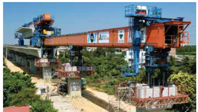
Figure 18. Stiff pier frames for dual-track box girders. Courtesy of VSL.
