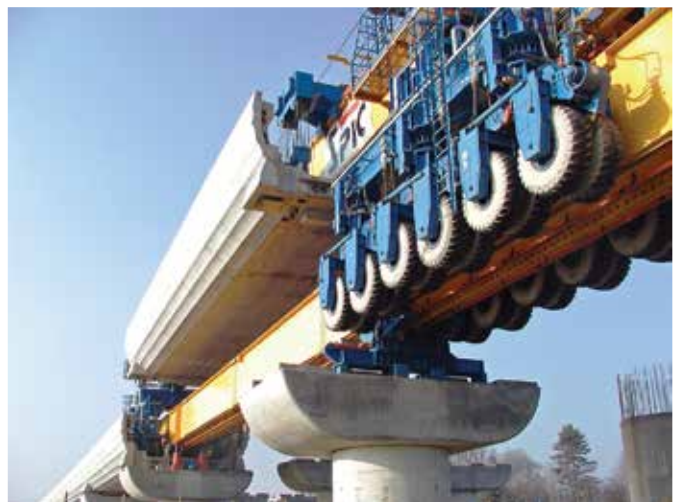
Figure 16. Portal carrier positioned for beam lowering.
