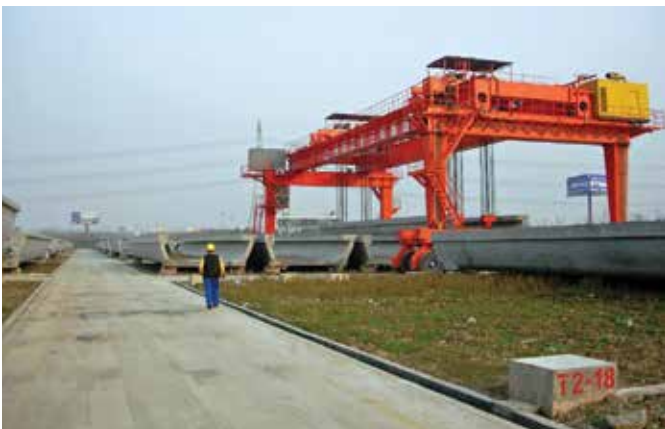
Figure 3. Large-scale storage of single-track U beams. Courtesy of Systra.
