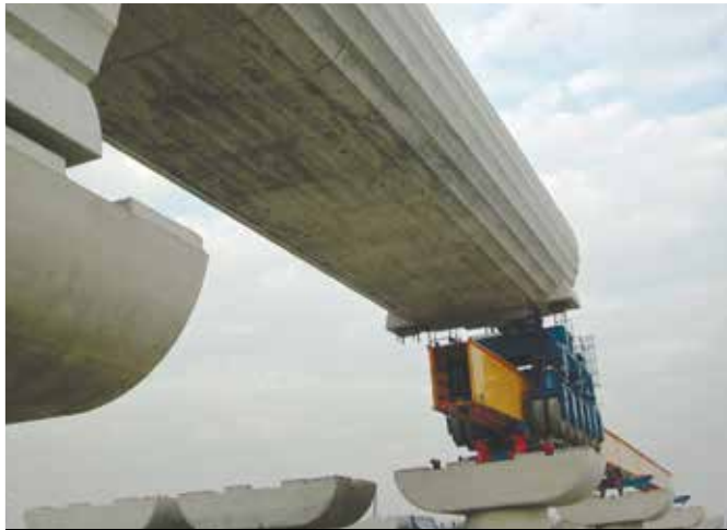
Figure 17. Repositioning the underbridge.
