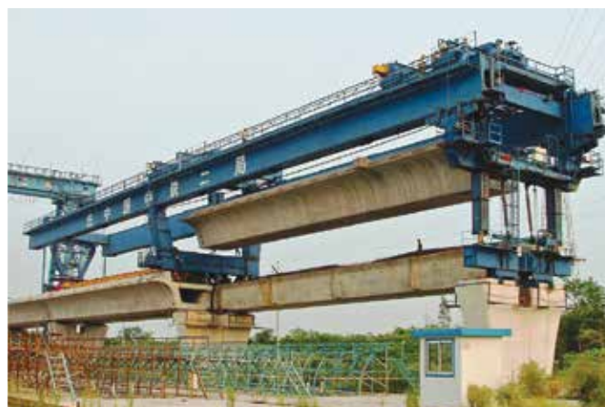
Figure 10. Twin-girder 2.3-span launcher for 32.7 m (107 ft), 4000 kN (900 kip) single-track box girders. Courtesy of BWM.
