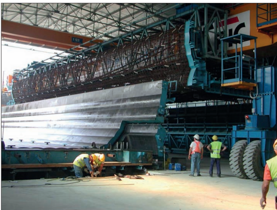
Fig. 2: Placing of the prefabricated cage into the casting cell
