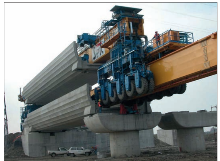
Fig. 6: Wheeled carrier advancing along the underbridge
