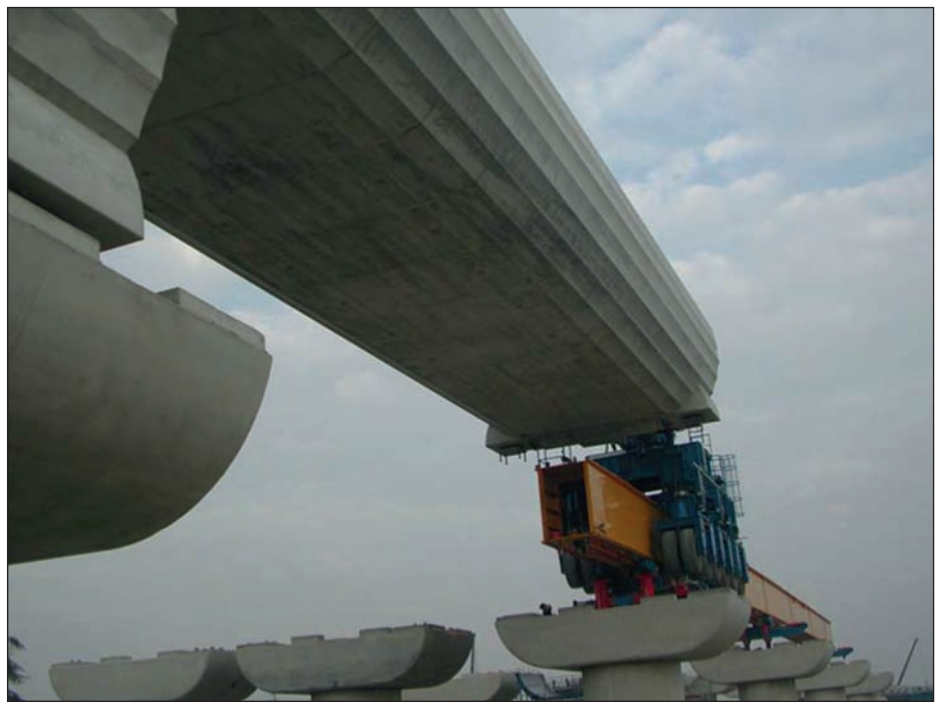
Fig. 7: Launching of underbridge clears the span lowering area
