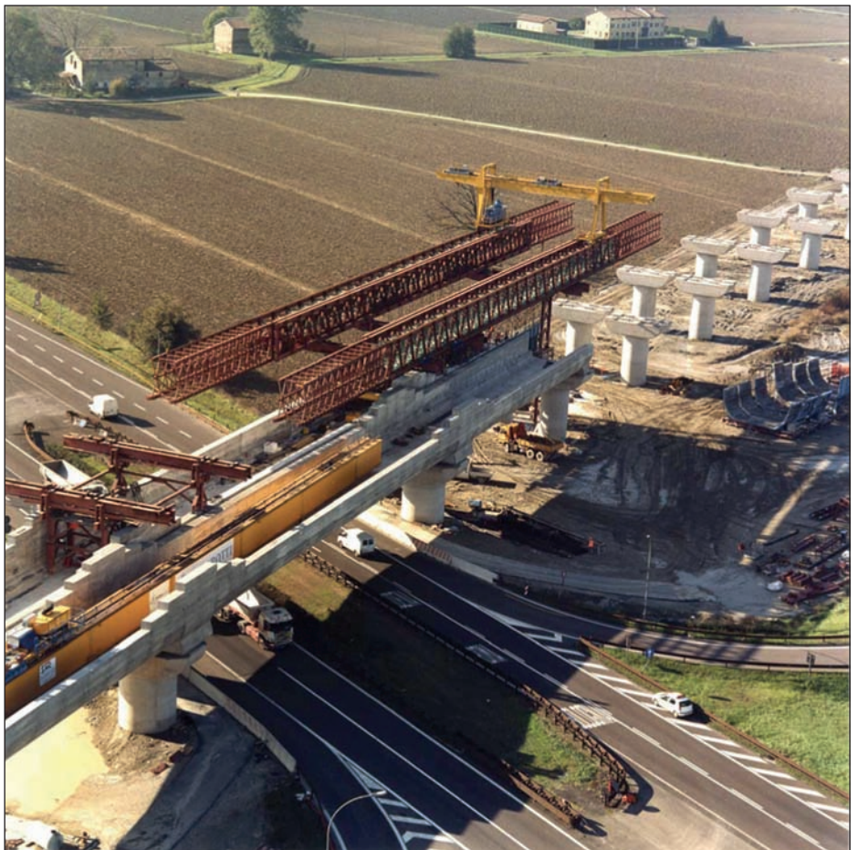
Fig. 8: Main MSS over Brenner Highway
