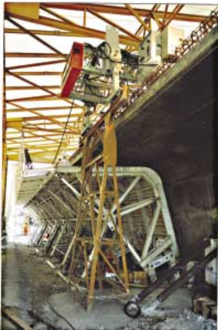
Fig. 10: Monolithic steel frame formwork (author).
