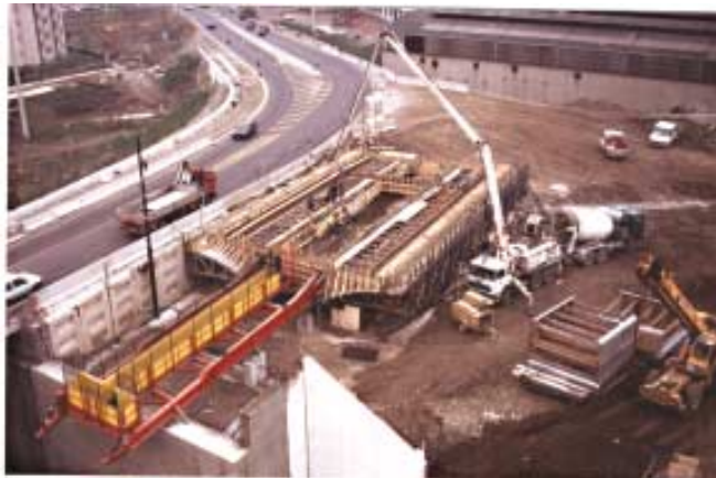
Fig. 9: Two-phase casting in a single formwork (author).
