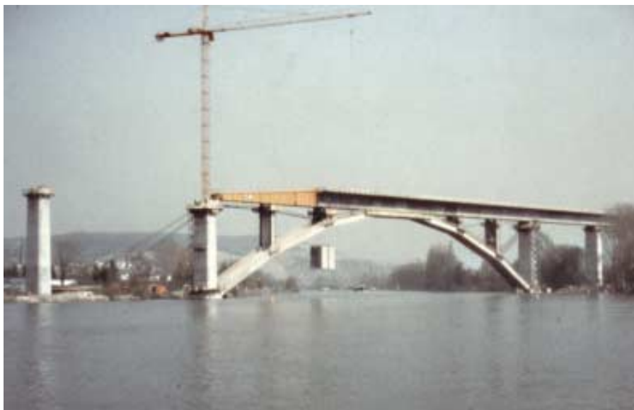
Fig. 14: Temporary balancing of launch stresses with cable-stays and counterweights (courtesy IIC).
