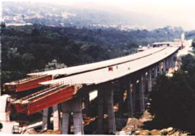
Fig. 12: Twin launching results in optimum labor rotation (author).
