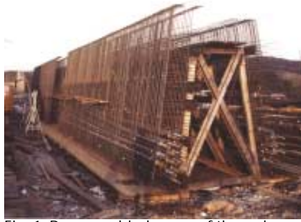
Fig. 1: Preassembled cages of the webs (author).
