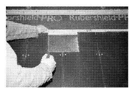
STEP 4: RE-POSITION SLATES AND FIX SECURELY. CAREFULLY CUT BATTEN FROM BETWEEN THE REMOVED SECTION OF SLATE.
