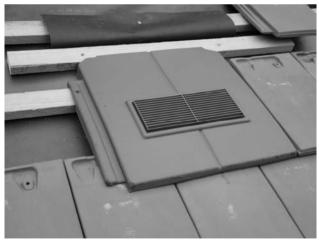
Position tile and secure through extended weather bar on the vent, as shown. Continue tiling.
