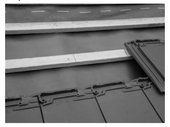
Determine a clear space between rafters to allow the Underbase of the vent to sit between.
