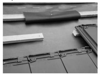
A hole in the felt will need to be cut. Protect this hole by inserting a section of felt at the nearest lap as shown. Wide enough to span beyond the hole
