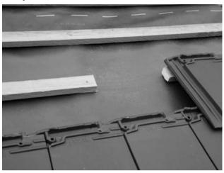
Where the underbase needs to locate, remove a Section of batten 270mm wide.
