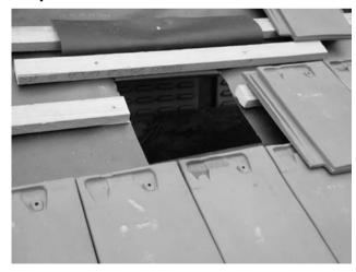
Carefully cut away felt, turning resulting flaps of felt outwards. Insert a support batten 130mm top to top to support the head of the vent.
