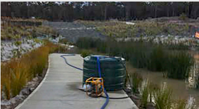
Dam water recirculation using pumps and a 1,000 litre tank
