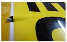
The hole is made using a Dremel drill and adjusted with a file
