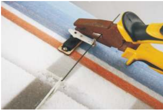
17. Use the pinchers to cut off the superfluous steel wire.
