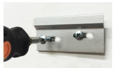
First, attach the two brackets to the wall. You an slide the frame so you are free to place the brackets as much as 20-40cm from the corners.
