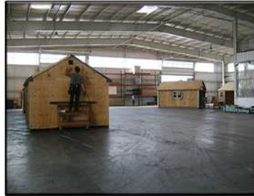
2) Amish Assemble The Building
