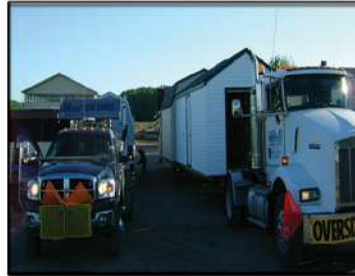
3) Building Is Loaded On Delivery Truck
