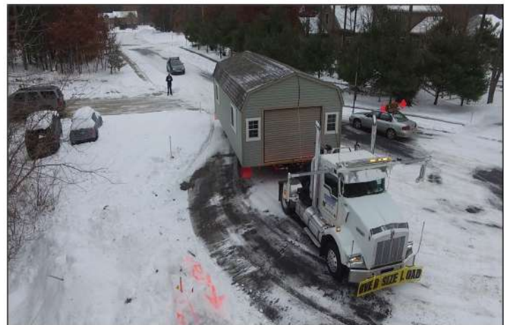
Winter Delivery - (Snow Must Be Cleared To Building Site)
