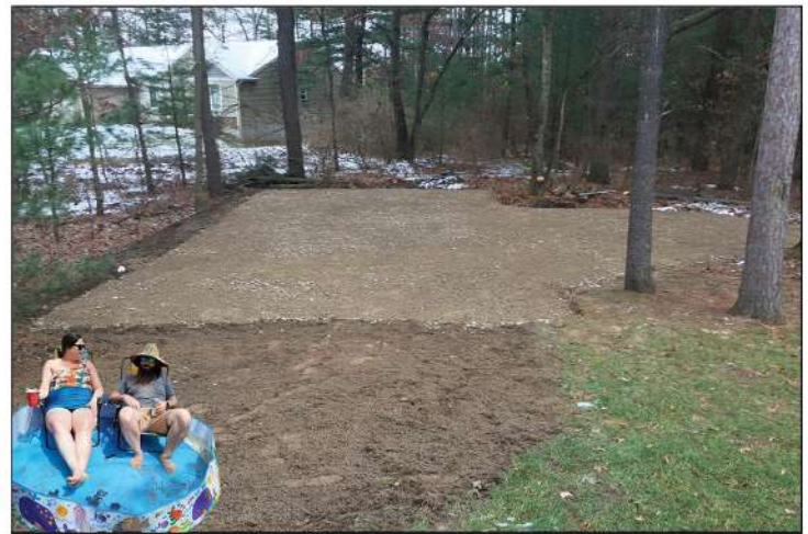
Crushed Stone Pad With Room For Fire Pit & Seating
