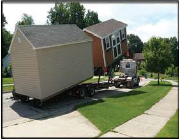
5) Hydraulic Trailer Unloads Building
