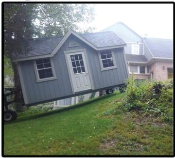
All of our buildings are delivered fully built and ready to use. We have specialized trucks and trailers equipped with a Mule Delivery System that allows us to maneuver the building to the shed pad with minimal impact on your lawn. The buildings can be placed directly on the grass but it is recommended to prep your site with 4"-6" of crushed stone to create a solid level base with good drainage.
