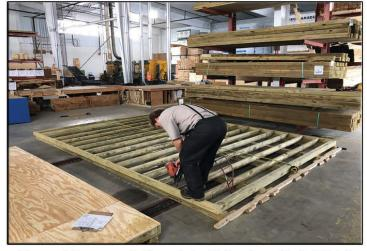
Treated Runners & Floor Joist Being Installed 12" OC
