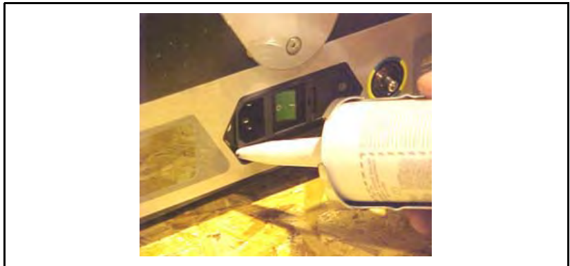
Figure 5-6. Seal Cover Around Power Inlet
