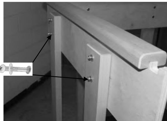
Figure 8: Straight Handrails attached
