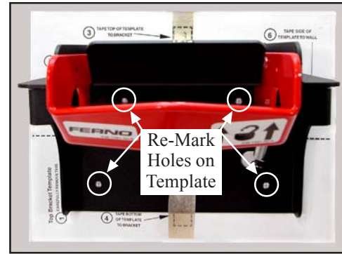
Figure 6 - Re-mark Holes on Top Template
