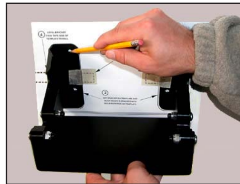
Figure 3 - Re-marking Holes on Template
