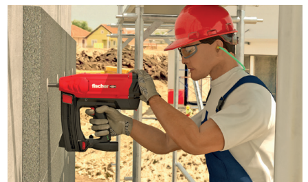
The special EWI-nose for the FGC 100 enables fixings of insulation systems
