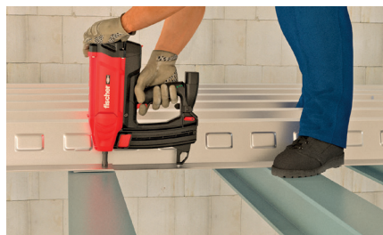
For temporary tacking of composite deck to steel beams
