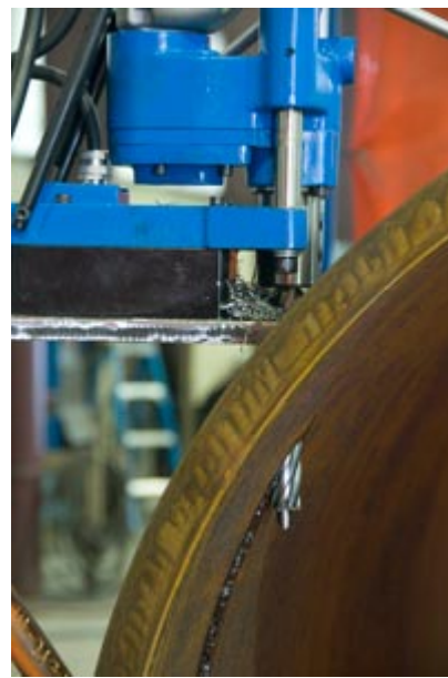
Hougen Rotabroach® Cutter after it has drilled completely through the side wall of a pressure vessel.
