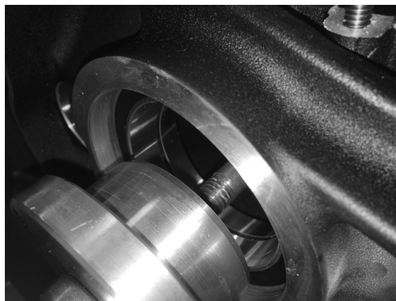
FIGURE 15 | TAPERED BEARING ADAPTER VISUAL INSPECTION
