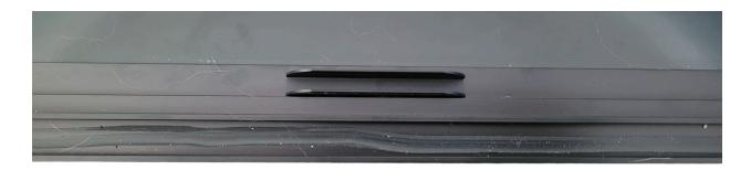
Step 6: Insert the Thin Rubber Door Strip (Part I) into the bottom glass door tracks. Insert by putting the strip in sideways and then allowing it to fall into place.
