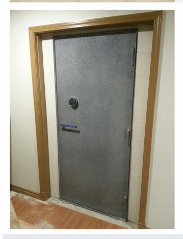
Now that the frame is fitting good and the door is opening and closing properly, go ahead and fill the gap between the frame and cement wall, which should be about 5/8" to 3/4" with high PSI mortar. Let it cure, then remove the wedges and fill in the wedge gaps with mortar. Test again to see if the door open and closes properly. Finish installing the rest of the anchor studs at this point. If you need anymore tips, please give us a call. 800-262-0023
