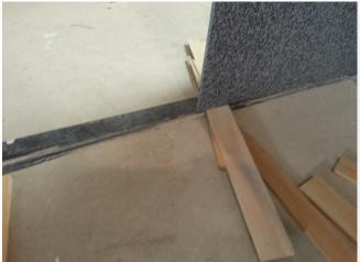
Once open the door will need support on the outside corner to help hold it up and to move frame back into the marked position in the cement rough opening.
