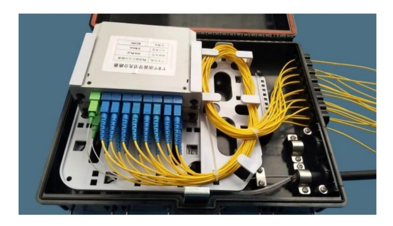
6. Fix the case with expansion screw, or hold on the pole with hose clamp, and the installation is completed.
