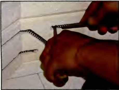
Inserting element into brick groove
