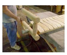
1. Attach both swing arm assemblies to swing seat. Align the two doweled ends of swing seat with the two holes in the swing arm assembly. Tap arms into place using rubber mallet or hammer. If using a hammer, be sure to pad impact area to avoid damage to the product.
