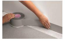
4. Cut suitable PVC cove former at least 20 x 20 mm (0.8" x 0.8") exactly matched and mitered. Cut 2 cm (0.8") of the release paper of Remur 95 at the lower edge and remove.
