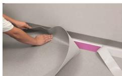
9. Fold Covering down from the wall and pull off release paper. Press floor covering to cove former and fold up or roll firmly onto the wall.
