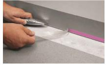
Apply cleaned PVC cove former from the corner. Press down onto Remur 95 section by section without stretching or pulling
