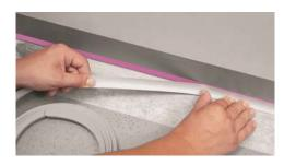
Apply Remur 95 to the floor from the edge of the installed floor covering and rub down. The PVC former will be slightly overlapping. Install Remur 95 to butt in corner area
