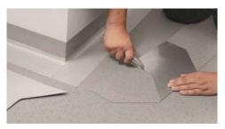
8. Pull off the release paper from the Remur 95 adhering to the floor. Start to install floor covering. Rub down or roll down firmly on the floor.
