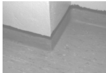
Fig. 3.6.1. Hot air Puttied Inside/Outside Corner
