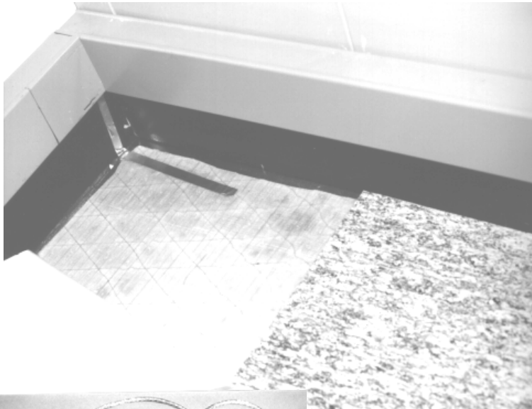
Photo 2.2.3 Grounding Plate
