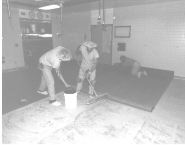
Fig. 3.4.2.1 Lay Out Oversize Sheets And Broom Clean
