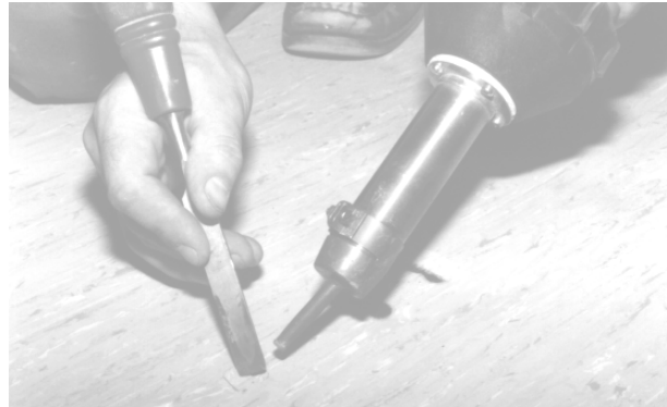
Fig. 8.2. Using A Tool To Heat-Putty Insert a Section of New Flooring
