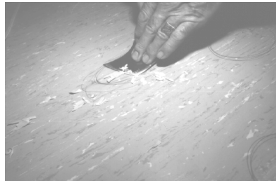
Fig. 8.4. After Cooling, trim excess repair piece flush with half moon knife and wood scraper.
