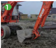
1 perform the excavation works
