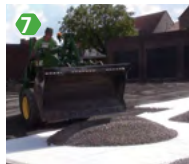
7 placing the gravel
