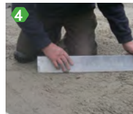
4 levelling the levelling layer
