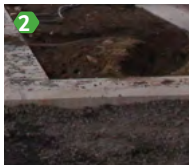
2 installing the borders
