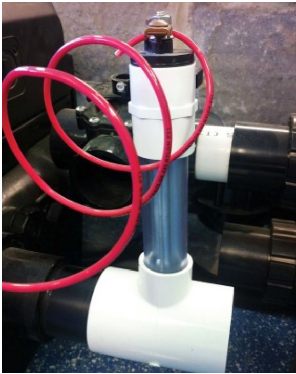
[4] An inline sacrificial anode installed on a pool system.
