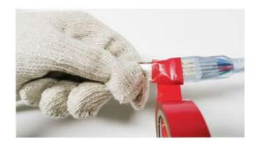
5). Use Electrical tape or shrink tube to double sealed.
