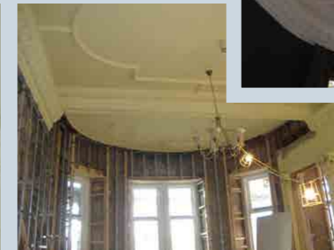
Dalziel Drive, Pollockshields: Again a very typical job for us, reinstating the cornice which was lost during rot works. Note the seamless transition from new to existing cornice, which is the standard of workmanship we pride ourselves in.
