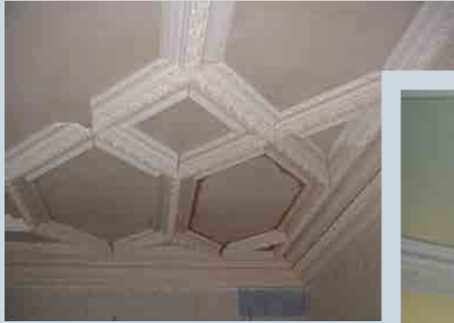
The Garrison, Millport: This ceiling was completely lost after lying derelict for years. Luckily samples of the cornice and ceiling panel moulding were retained for moulding purposes, but the general ceiling layout, and in particular the entire centre rose, were recreated purely from photographic records.
