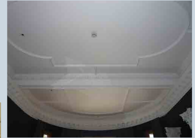
Dalziel Drive, Pollockshields: Again a very typical job for us, reinstating the cornice which was lost during rot works. Note the seamless transition from new to existing cornice, which is the standard of workmanship we pride ourselves in.
