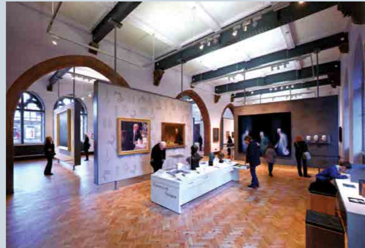
Scottish National Portrait Gallery: This major restoration project required the skills of our tradesmen on site for a total of 14 months, repairing and installing over 1000m of cornice work. This was part of a 3 year project undertaken by BAM construction.
