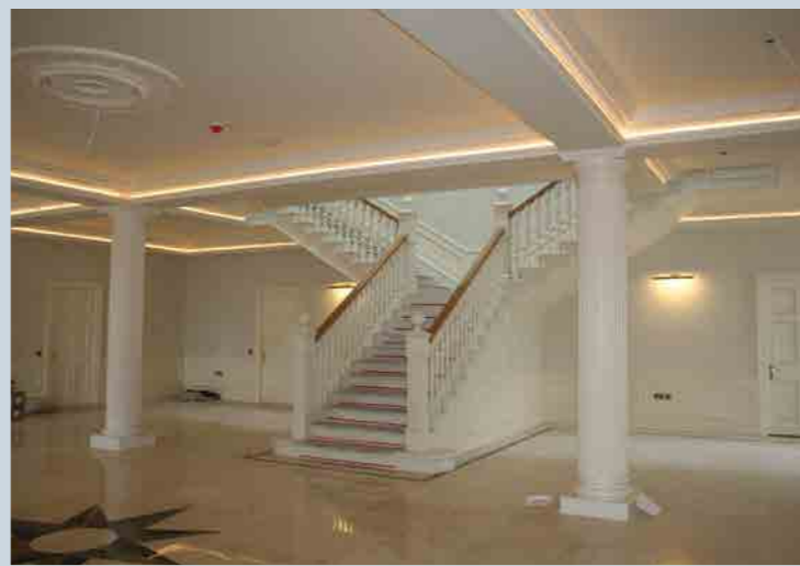
Columns – Private residence: As well as installing the very effective lighting trough cornice detail, the fluted Doric columns were entirely custom made in order to produce a product large enough to encase the structural steel columns.
