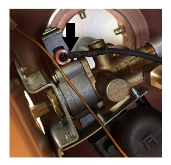
Remove the ignition wire from the control housing.
