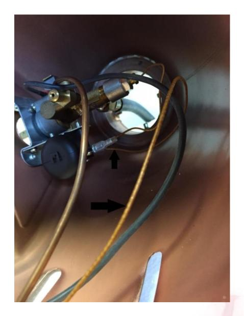
Remove the thermocouple wire that is connected to the tilt switch.
