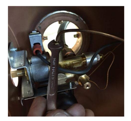
Remove the gas line with an 8mm wrench.
