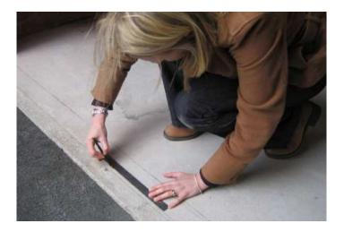
Open the door and mark a line along the front edge of the seal. Remove the seal and mark two parallel lines approximately 10mm inside the existing lines. Then mark a zigzag line in the middle of them.
