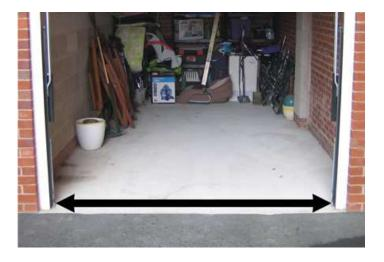
Open the garage door and measure the overall width of the opening. Allow approximately 40mm (1 1/2") overhang to allow the floor seal to be notched back around the door frame or side tracks. Then cut the length to size.
