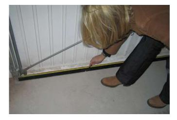
From inside the garage, with the door closed, push the seal up to the back of the door with the hump touching the door, or as tight as it will go whilst still ensuring the door will close and lock in place. If necessary, notch the ends of the threshold back further to create a tight seal. Mark along the back edge of the floor seal with a pencil or suitable marker.
