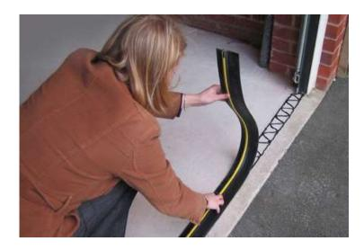
Begin from one end. Place the seal on top the adhesive and press firmly downwards. Continue along the rest of the seal, ensuring good contact at all points. Remove any excess adhesive from the sides with a cloth. **Note:** Once fitted allow 24 hours before driving over the threshold seal. It is also recommended to test the installation using a bucket of water of hosepipe to check for water ingress.
