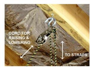
Step 7: Attach the straps to the object being raised. Installation is now complete.
