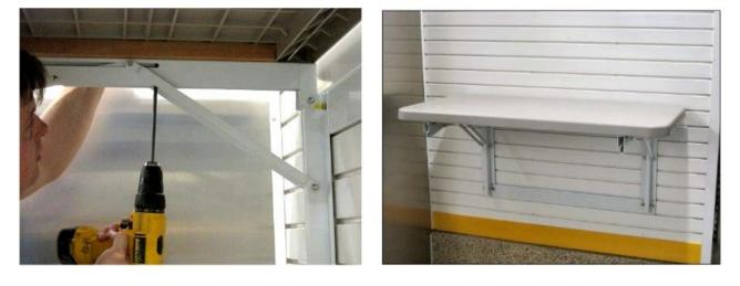
Step 7: With the supplied 1" screw, fasten through the rear 2 holes on each bracket into the stiffener previously installed on the table top.
