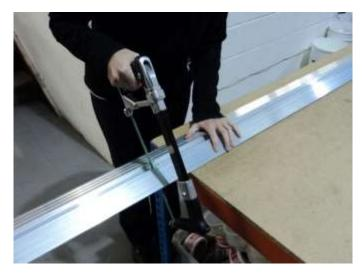
Cut the aluminium sections(s) and the two bottom rubber seals to the size of the aperture.
