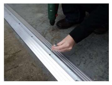
Apply pressure on the Threshold Seal by standing on it. This will compress the two side seals. Then tighten the fixing fully.
