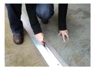
**(Position A)** Position the Threshold Seal in line with the centre of the door so the door will close on the black and yellow cap that runs along the centre of the aluminum section(s).
