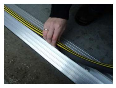
Clean out the channel with a clean cloth to remove excess dirt. Starting from one end of the threshold, pinch the legs of the rubber black and yellow inset and push it in to the top of the threshold until it 'snaps into place'. Continue this process with the remainder of the threshold, taking care to ensure that it is firmly pushed down.
