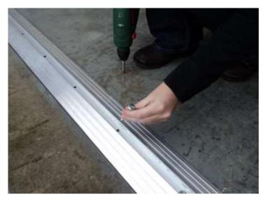
Using an electric screwdriver with the screwdriver bit T30, tighten the fixing until the screw is approximately 5 mm from going all the way in.
