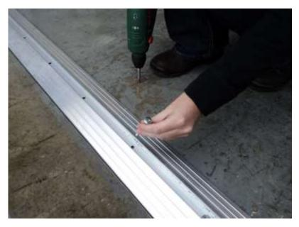
Re-position the Threshold Seal so that the pre-drilled holes in the aluminum seal coincide with the holes drilled in the concrete floor. Starting from one end, place each fixing screw into a hole. There is no need to use plugs as the fixings have a cut thread design that enables them to be drilled into concrete.
