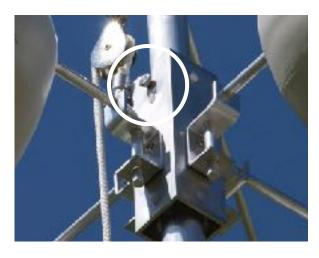
Step 17) It's now time to raise your hub. Take hold of the end of the rope. Step back from the pole about 3 feet, and pull on the rope. Your hub will raise towards the top of the pipe. The notch in the hub will need to slide into the alignment pin, thereby locking the hub into the place. Hanging on to your rope and walk
